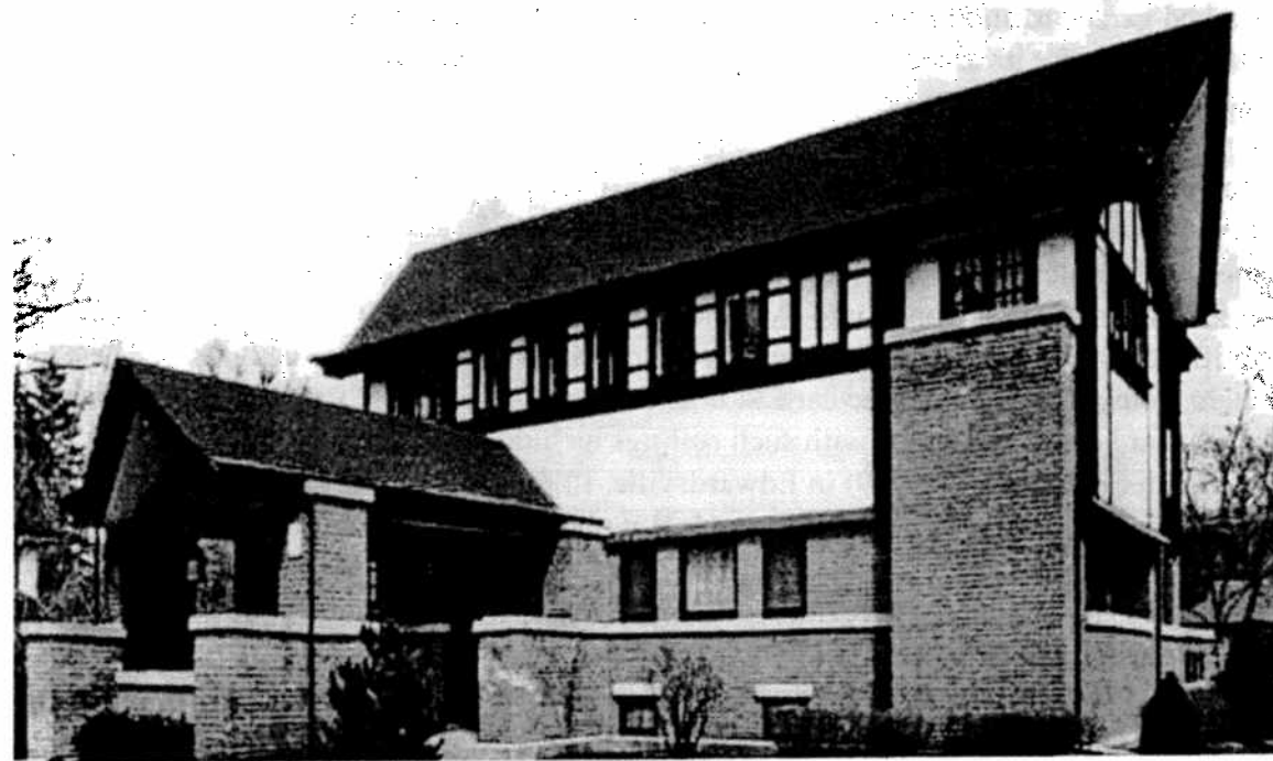
Top: Chicago's Robie House (1910), one of the seminal buildings of the Prairie style, designed by its acknowledged originator, Frank Lloyd Wright. Bottom: The Emery House in Elmhurst, designed in the Prairie style by Wright protegee Walter Burley Griffin. Note the house's vertical emphasis in marked contrast to the horizontality of the Robie House.
